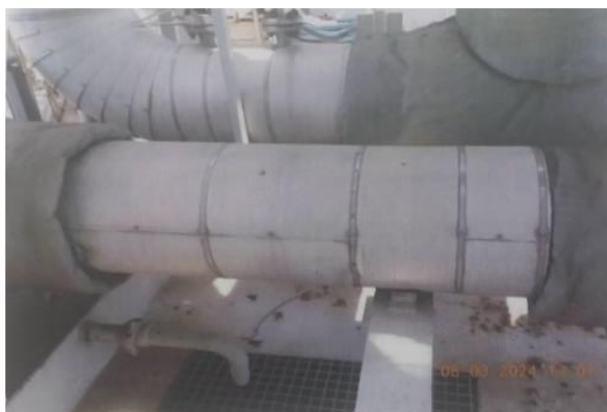
Fig. 2. Examples of PEC inspected insulated pipes
