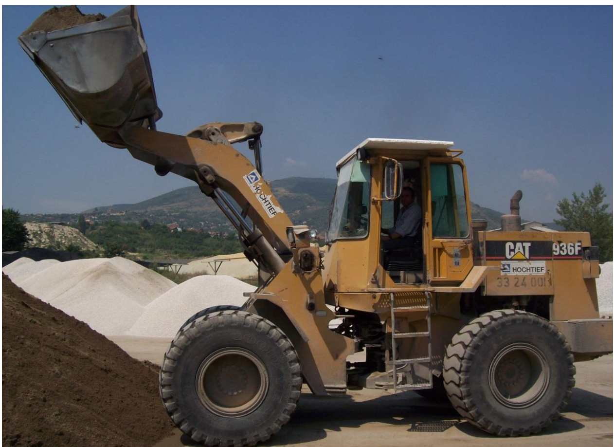
Fig. 6. Testing of a Z-kinematic loader in Skopje Cement industry “Titan”-Usje (Photo:J. Jančevski)
