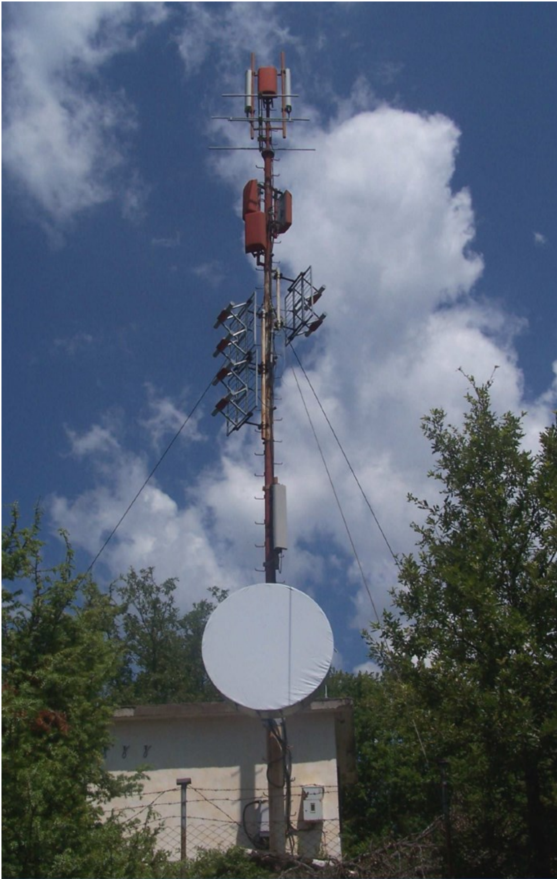
Fig. 1. Outline of the antenna mast before the disaster
