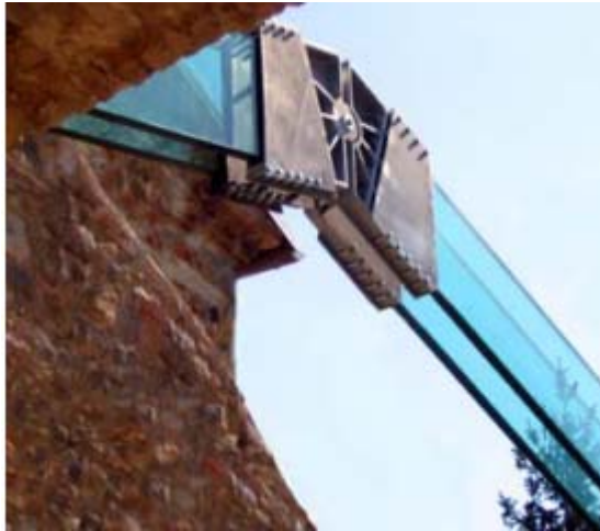
Fig. 4. CFRP reinforced glass beams [6]
