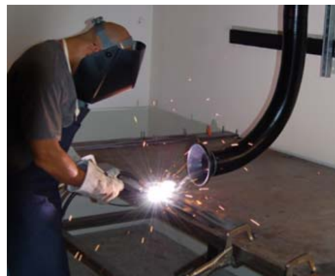
Fig. 3. Exhaust ventilation using welding Fume Extractor that is mounded on the wall.
