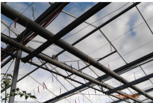
Fig. 3. High position of heating pipes
