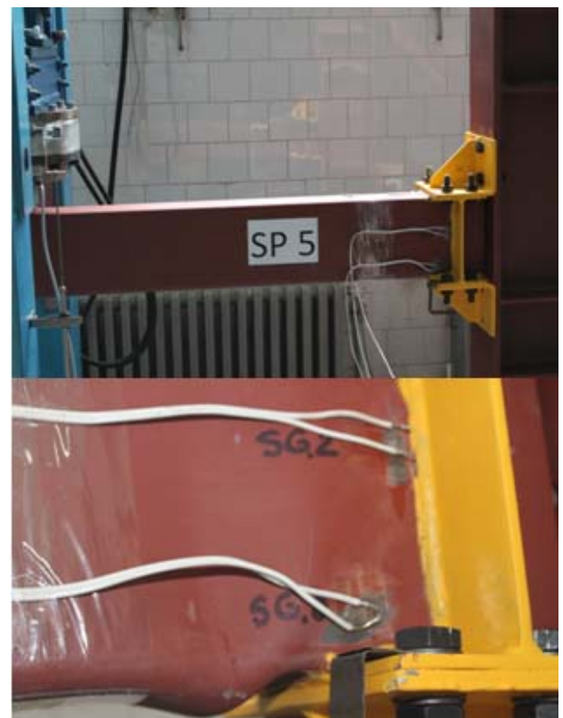
Fig. 17. SP5 model: Appearance of the plastic hinge (stability problem of buckling in the lower pressed part of the beam)
