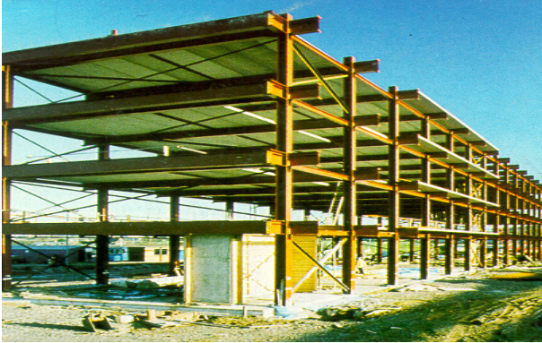
Fig. 1. High-rise parking building (under construction)
