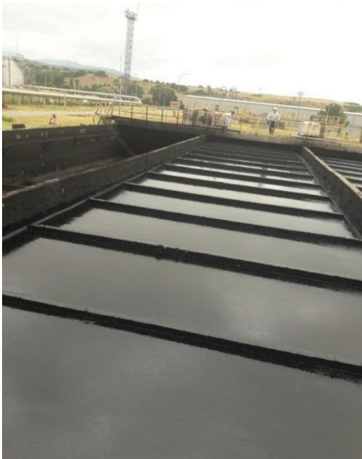
Fig. 5. Separation of the oil products
