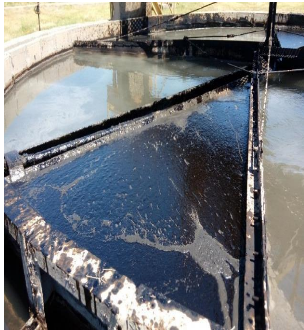
Fig. 6. Flotation upgrade of the biological part of the plant with nutrients
