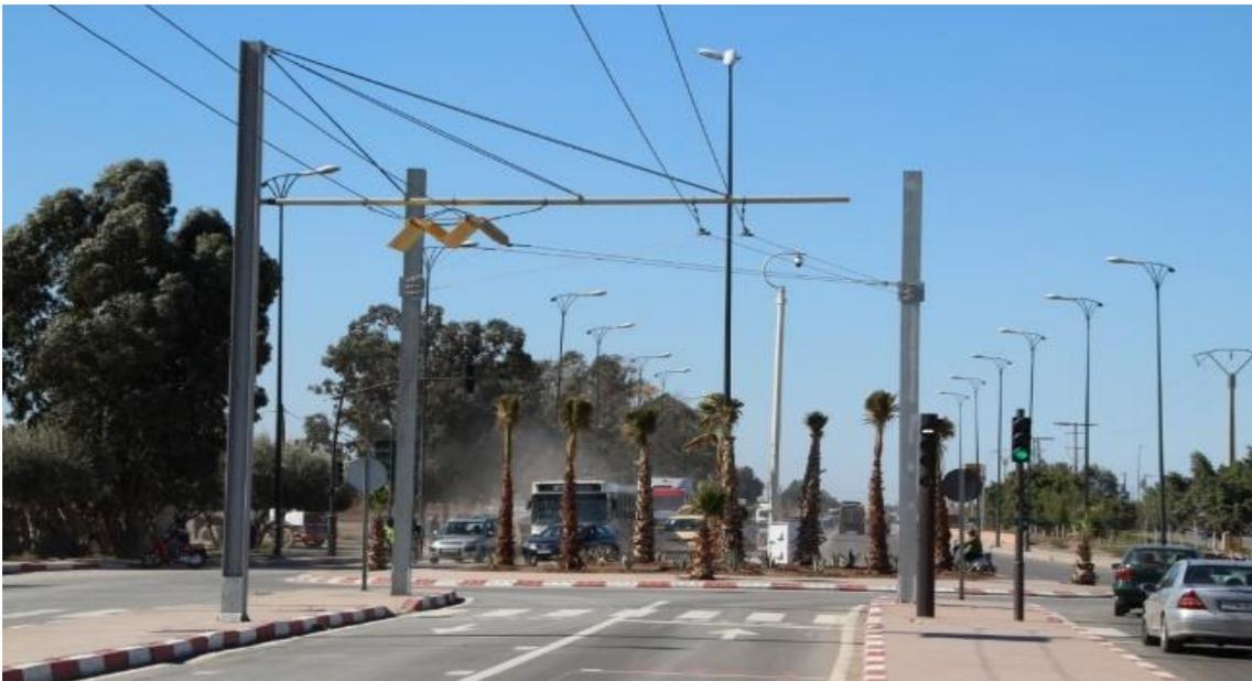
**Fig. 8.** The western end of the catenary section of Marrakesh's BRT system
